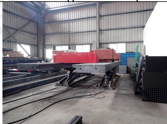
Photo "C" Loading test
